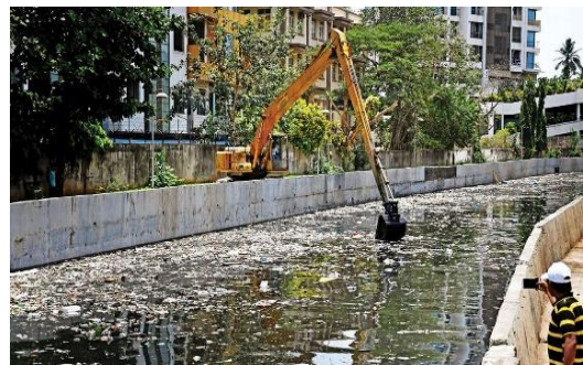
Figure 2. 2: Cleaning of drains in Mumbai
