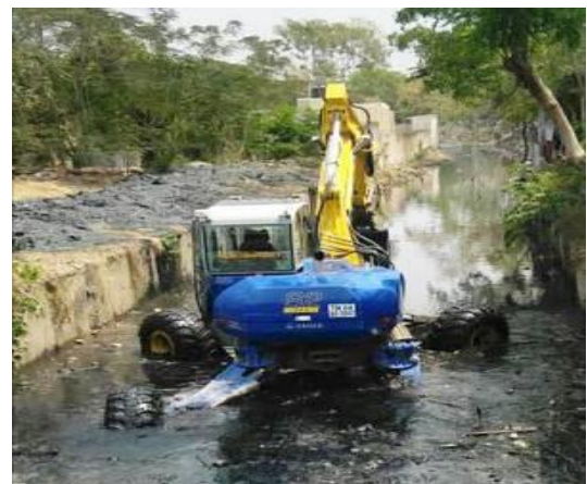
Figure 2. 3: Robotic Excavator in Chennai
