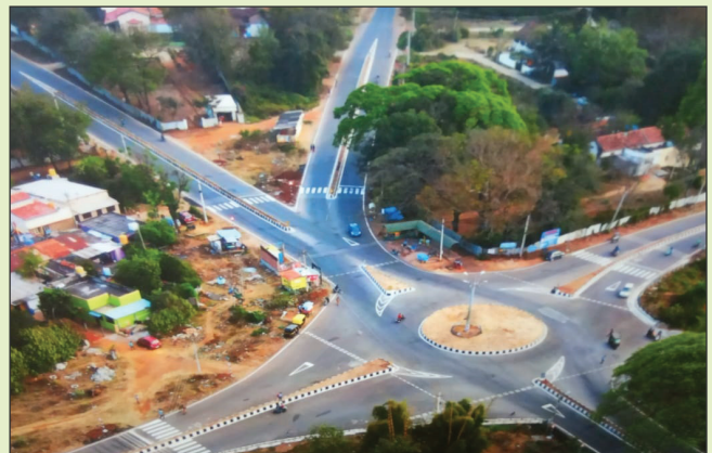
Road Safety Works on KGF State Fund Road near five light circle in Bangarpet Taluk, Kolar District.
