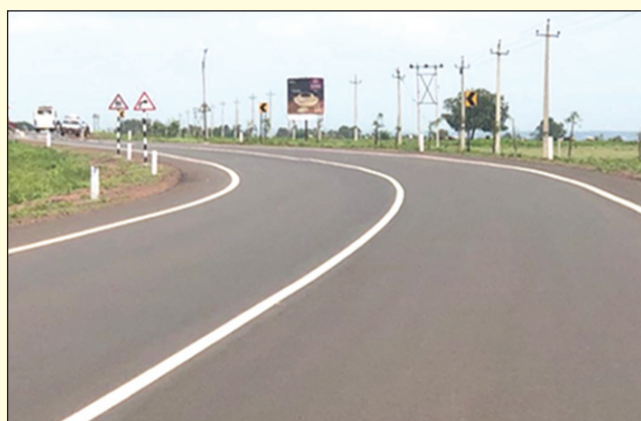
World Bank Co-Finance Project :- Bidar – Chincholi road (WCP-2)
