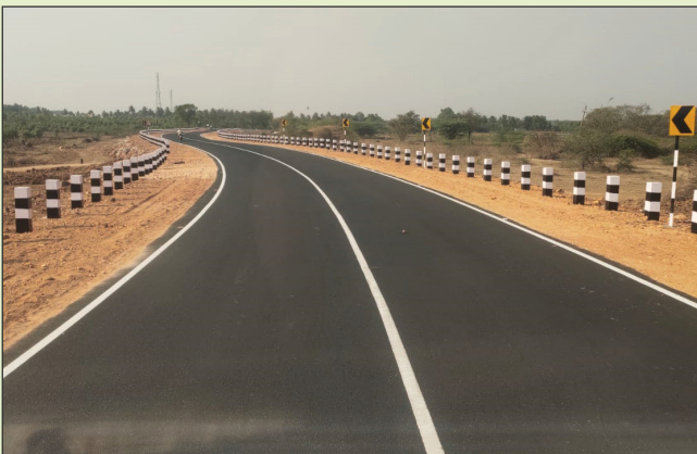
Road Safety work on Bangarapet Bagepalli Road (SH-15) from Ch. 21.20 to 21.60 km and 39.20 to 39.40 in Kolar Taluk, Kolar District
