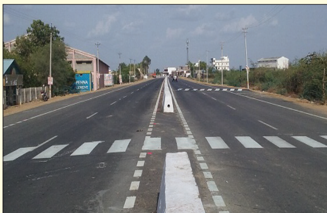
Improvements to Sindhanur - Kushtagi via Tavaragera Road (SH-30)
