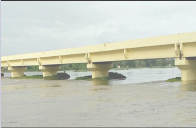
Bridge across Shimsha river near Vaidyanathapura
