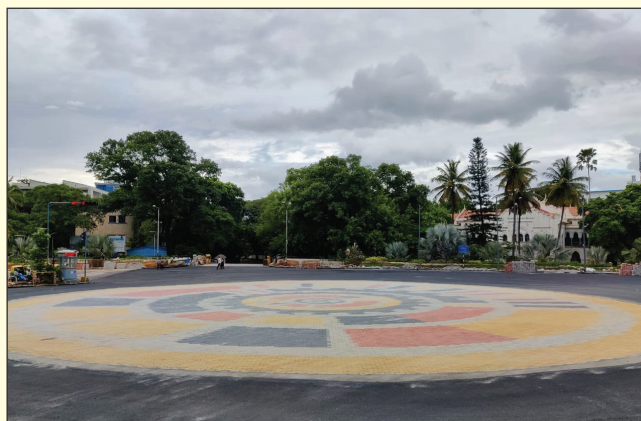
Development Works at K. R. Circle, Bengaluru
