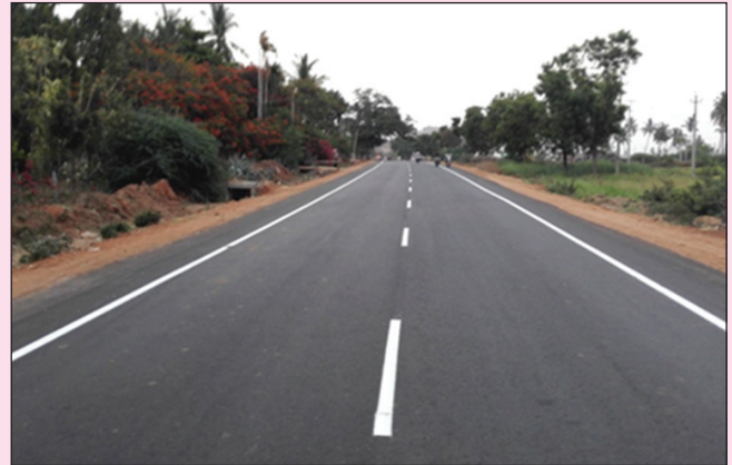
PPP- DBFOT- VGF (Toll) project: Ginigere- Gangavathi - Sindhanoor road
