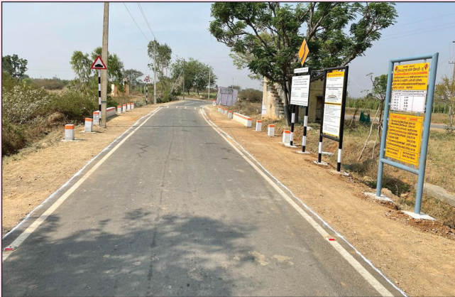
Nayakarahalli Hudukula road in Kolar District (PMGSY)
